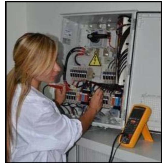
Insulation test @ 1,000V
